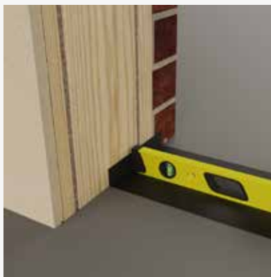
Ensure base under threshold is flat & level.
