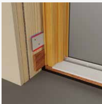
Temporary fixings to be installed into jambs – Once the door is in position fit temporary fixings to hold the frame in place. Check with a long spirit level that the frame sides are plumb and square.
