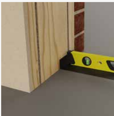
Ensure base under threshold is flat & level
