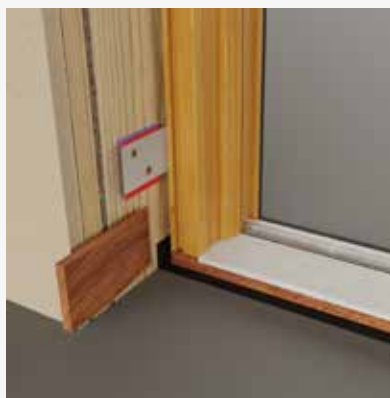
Remove wedges. Check levels and fixings.
