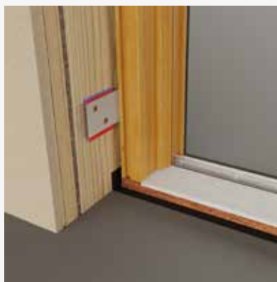
Refit the door. Fixings can be adjusted until the door operates smoothly. Check that there is an even clearance between the door and frame.
