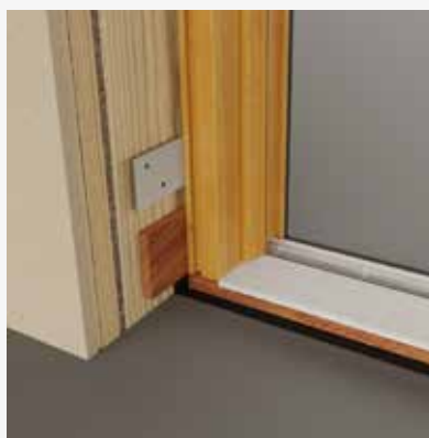
Secure with wedges. Wedge at the bottom of each side (opposing wedges from inside and outside) so the top can be adjusted without the bottom moving.
